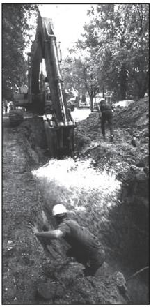
Several OSHA violations are present in this photo: no egress, no high-visibility clothing, accumation of water, and lack of a protection system such as sloping or trench box.
